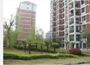
Ruian garden plot smart home engineer in Wuhan
